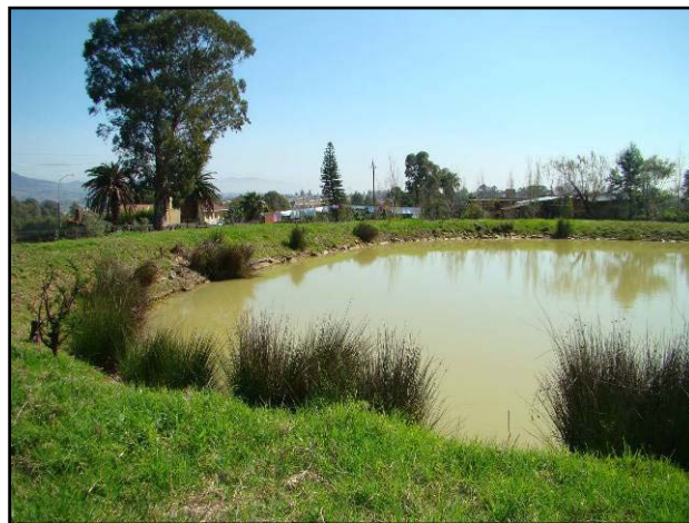
Plate 3: The earthen dam and farm worker's house in the background.
