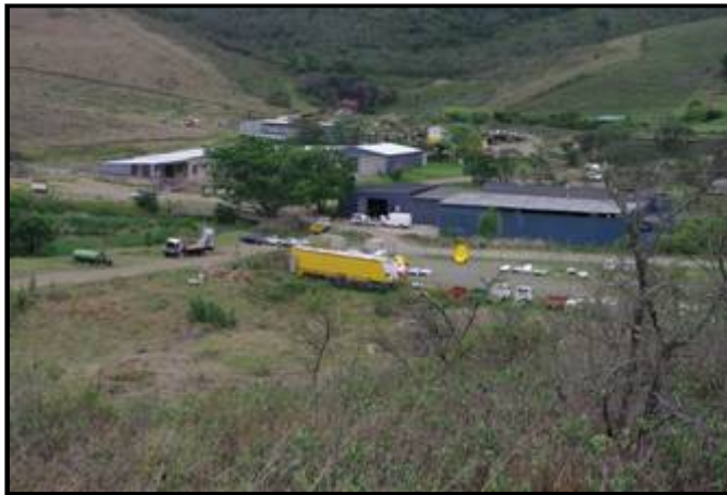
Figure 7: Close-up of the C1 infrastructure
