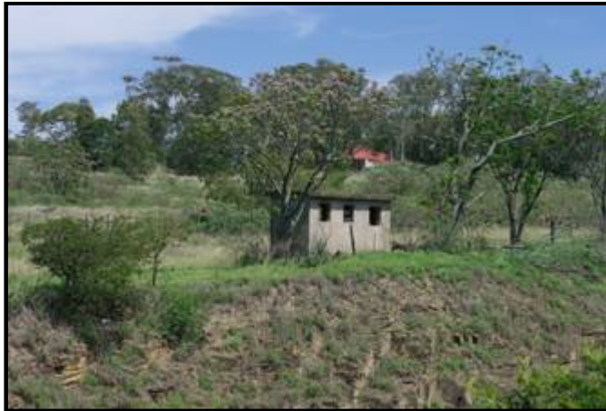
Figure 8: Recent structures situated in the vicinity of the C2 brick works
