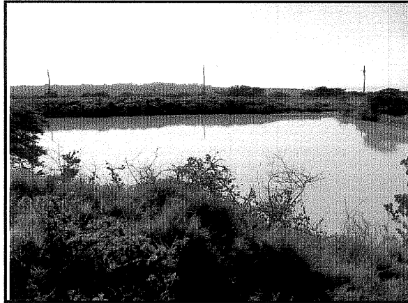
Figure 9: General view of Dam 1
