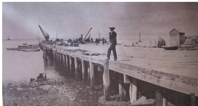
Figure 3: Photograph of the wooden jetty (Central jetty) at the end of Adderley Street c1902 (Picard 1969:118). The central jetty was constructed in the 1850s and became the central hub of harbour activities. In 1907 the jetty was extended to create a central pier and promenade. The pier was demolished in 1938 to make way for the Foreshore Reclamation Scheme (Patrick et al 2010).
