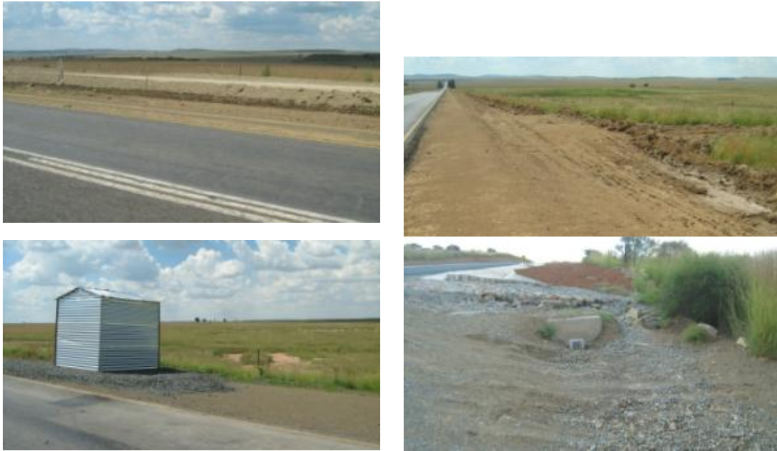
Figs 1-4. Extensive road works occurring between Smithfield and Reddersburg.
