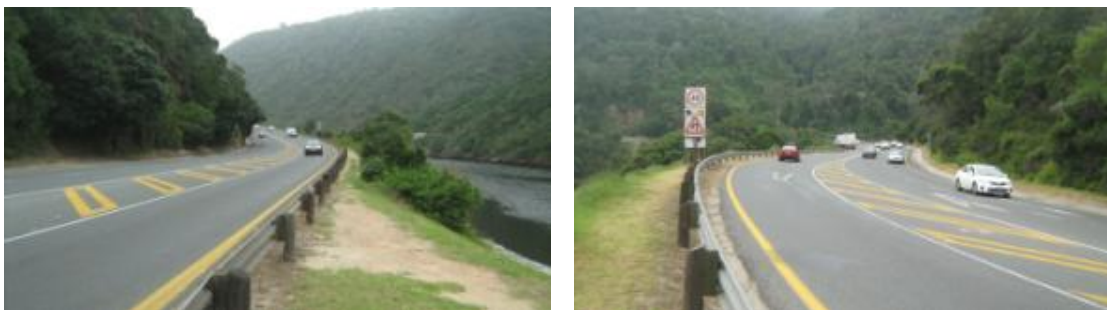
Figs 60-61. Views of the new road constructed in the Kaaimans Pass between George and Wilderness.
