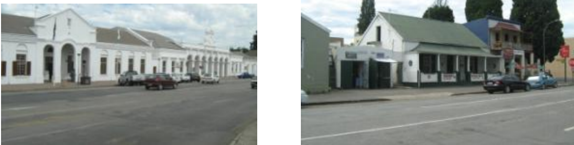
Figs 58-59. The town hall complex and library (left) and the declared national monument that is currently used as a doctor's surgery (right) situated in Cradock's main road.
