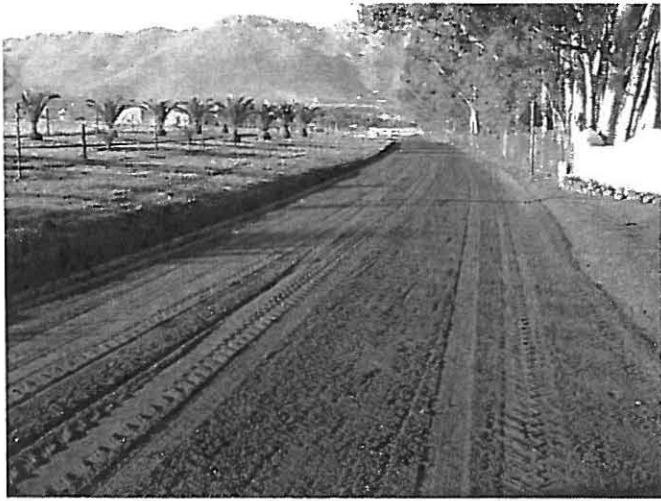
Figure 3. View of pipeline route facing east
