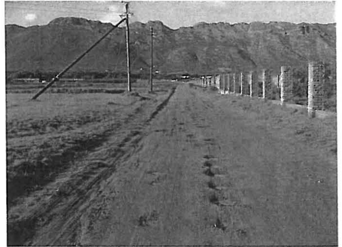
Figure 6. View of pipeline route facing east
