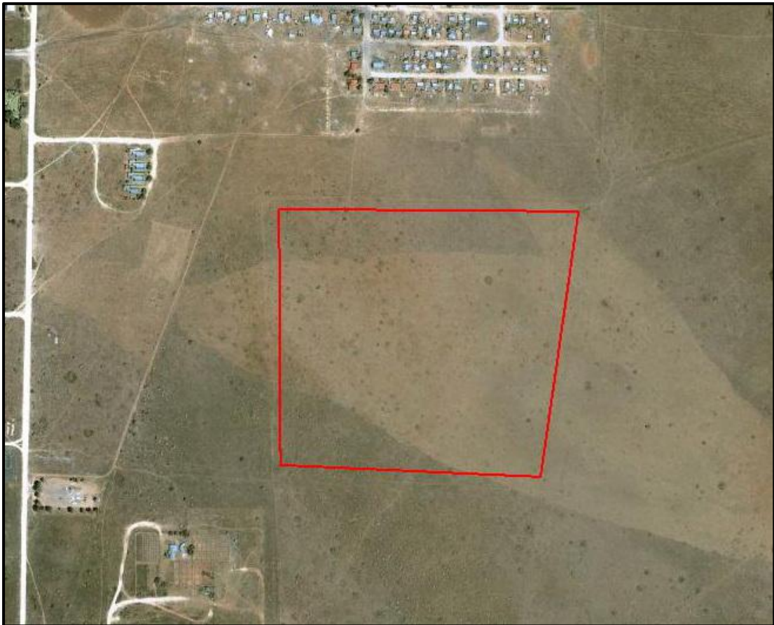
Fig. 14. Aerial view of the site showing a lack of natural as well as manmade features. (Photo: Google Earth)
