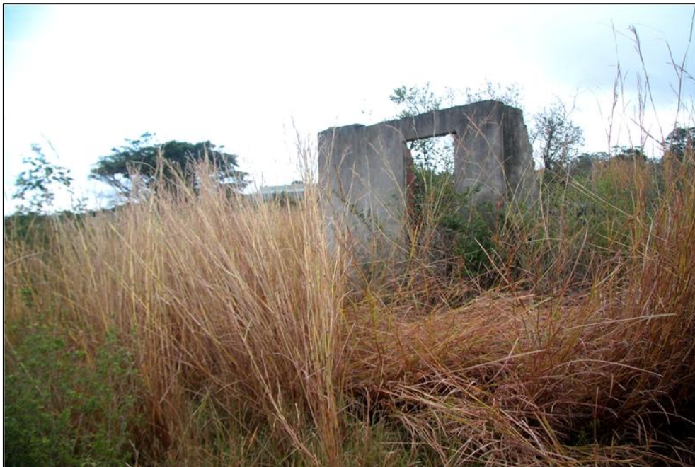
Figure 6-2: House ruins: remains of brick walling.
