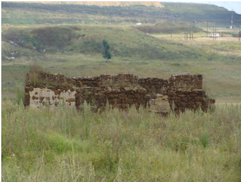
Figure 13 Ruin of a farm workers dwelling.
