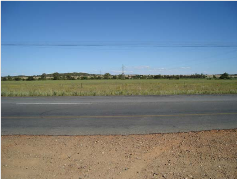
Fig.21 Point 19. Power line crossing N12.
