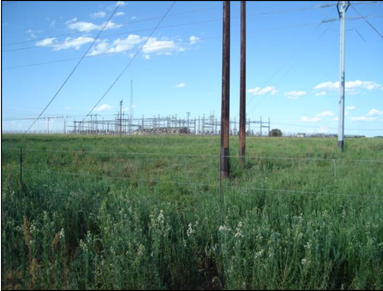
Fig.22 Point 22. Mercury Sub-Station between Orkney and Viljoenskroon.
