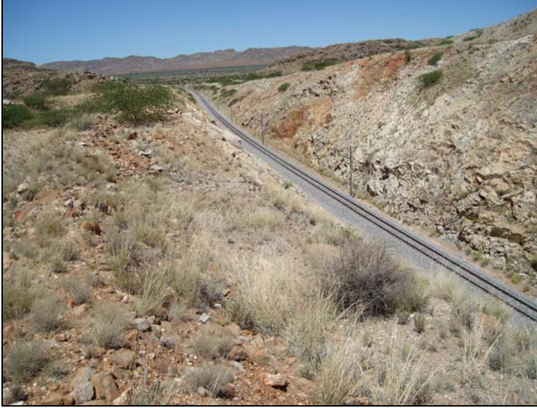
Fig.2 Point 2. The cutting for the railway line.
