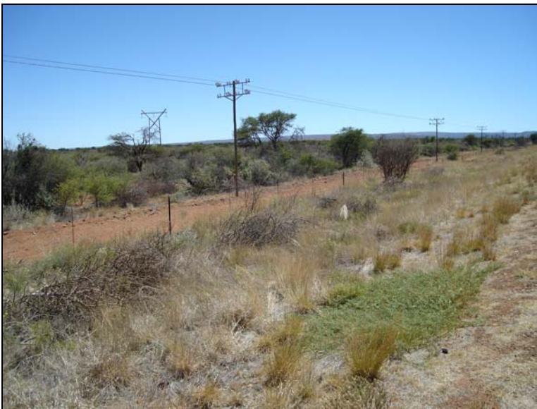
Fig.15 Point 7. Power line crossing the N14.
