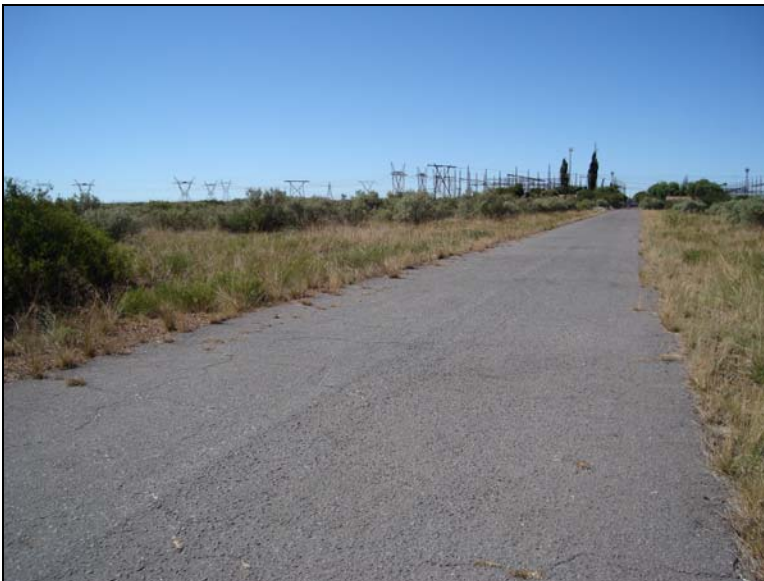
Fig.7 Point 12. Ferrum Sub-Station at Kathu (Map 1).
