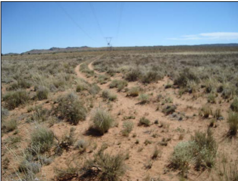
Fig.3 Point 4. General view at Pylon 373 (735km).
