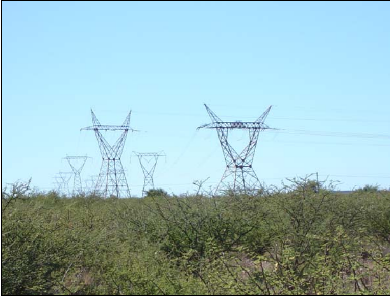
Fig.6 Point 10. The elbow in the power line
