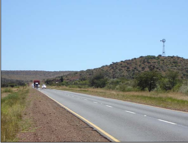
Fig.16 Point 8. The cutting at Red Sands on the N14.
