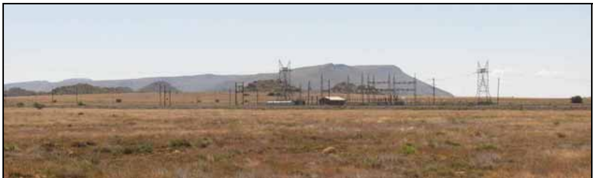
Plate 2: View to the east, toward the substation and railway line.
