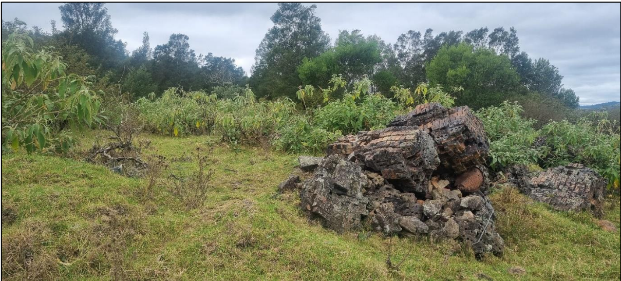
Figure 14. View of building material dumped within the proposed development area.
