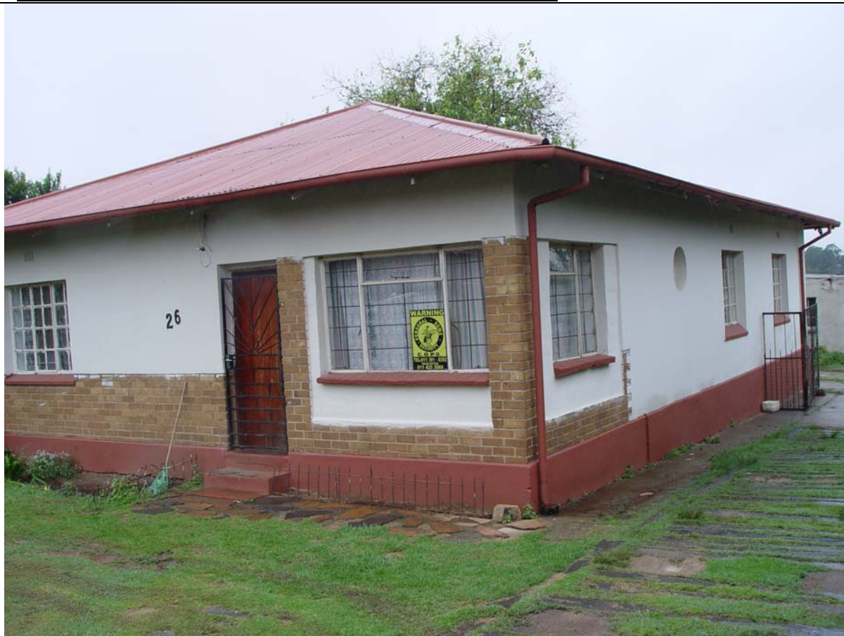
Figure 3: Multi-room brick house with corrugated iron roof.
