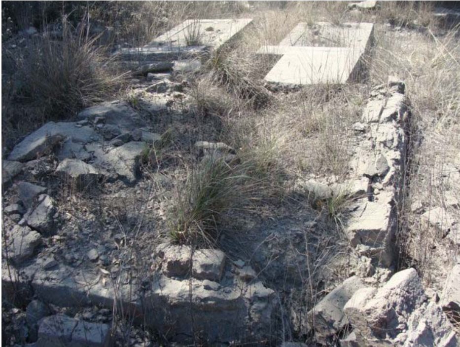
Figure 7 Some of the graves at site 1. Note the cracks and fallen headstones.
