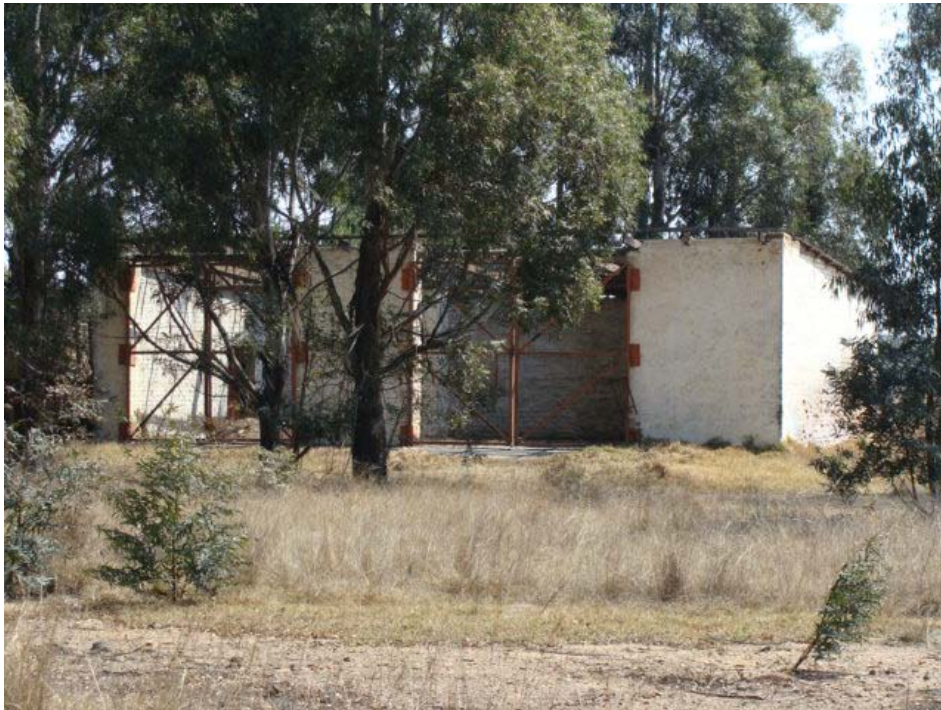
Figure 11 Storage building at site 2.
