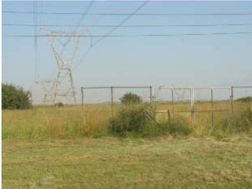
Figure 4: View of line taken from close to Glockner substation
