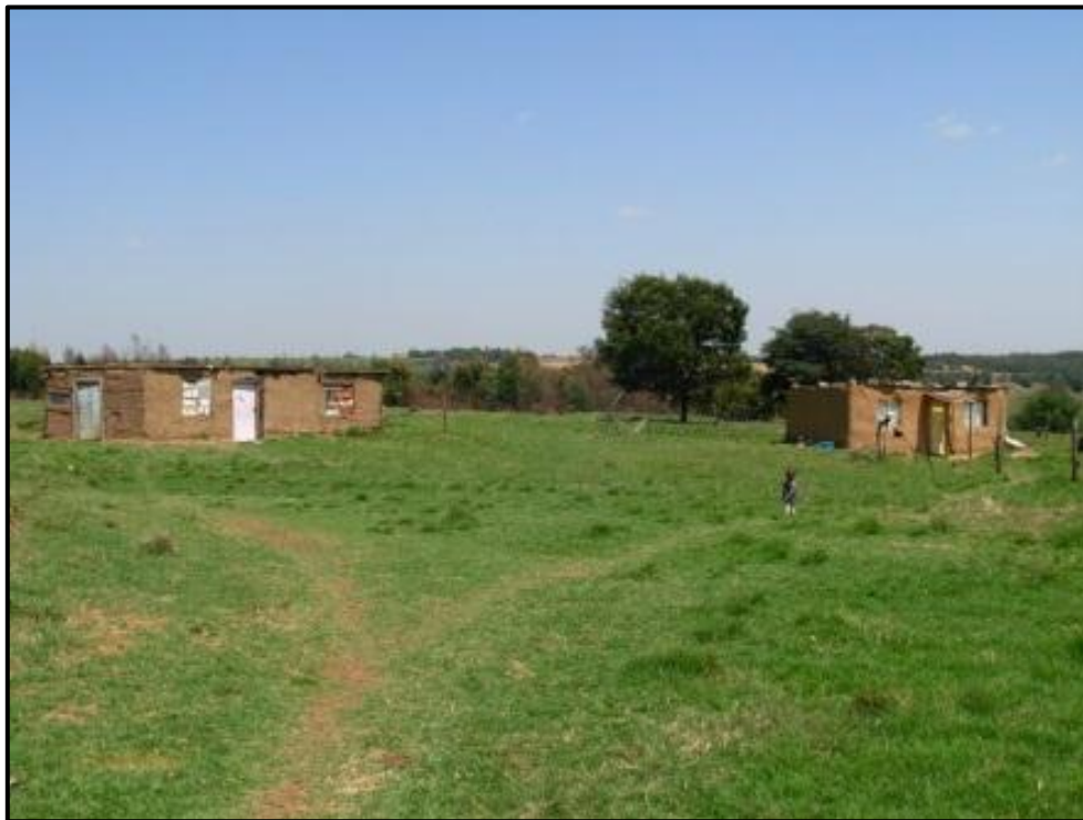
Figure 17 – Homestead with pole and daub structure
