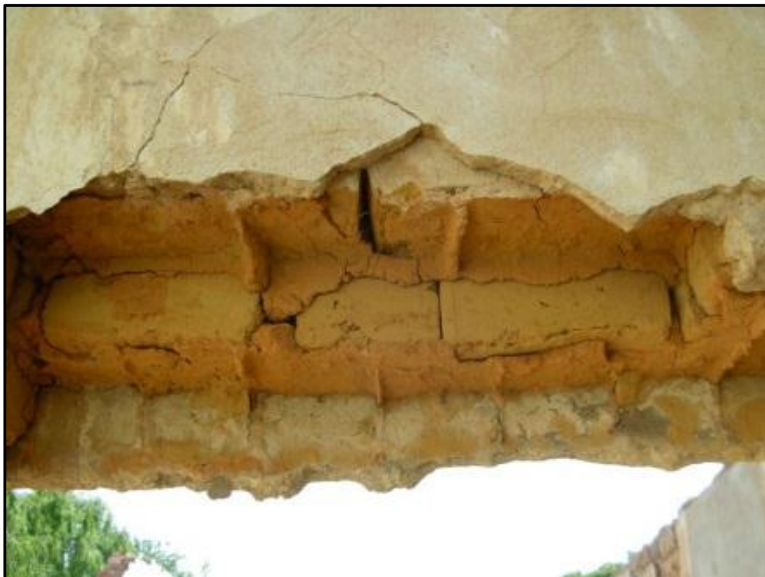
Figure 12 – Sun –baked bricks above lintel
