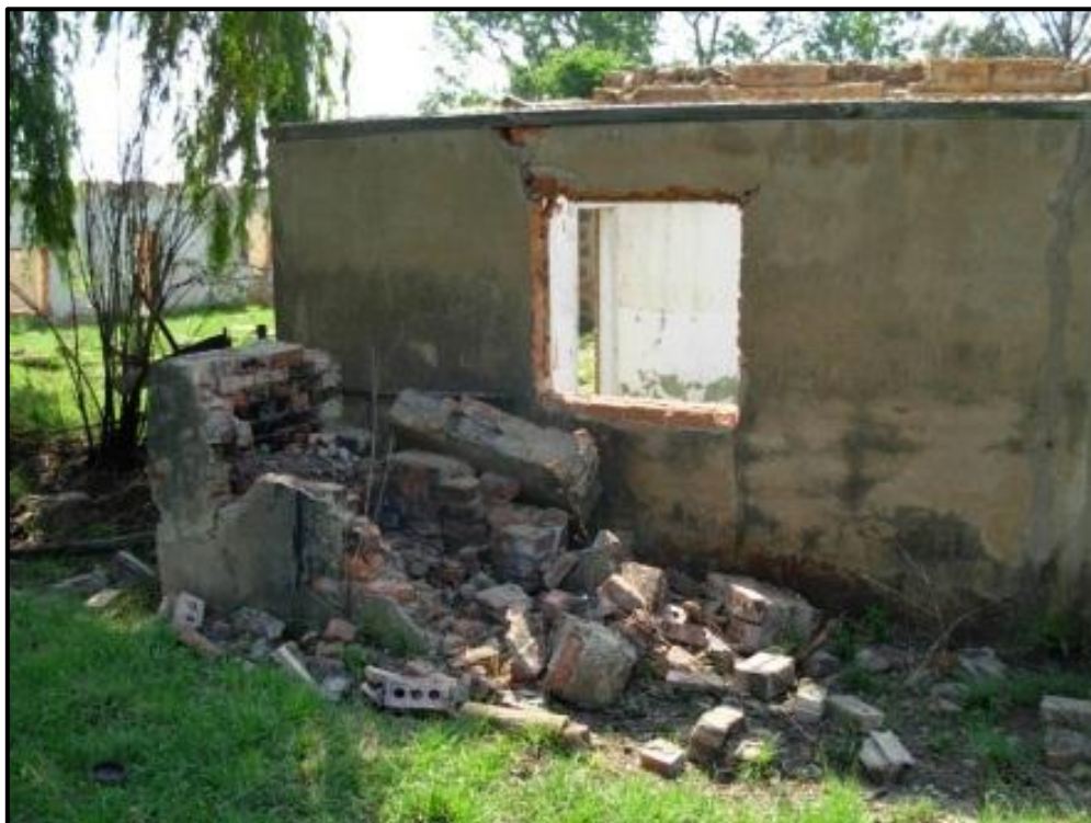
Figure 10 – Wood burning water heater
