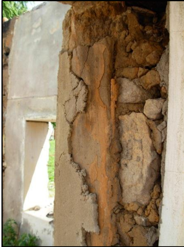
Figure 13 – Mud and cement plaster on in side of original structure
