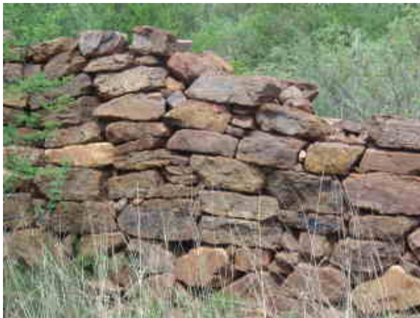
No. 2 Detail of well built stonewall
