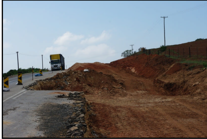
Figure 2: General view of the R72 Aurecon upgrading project in progress
