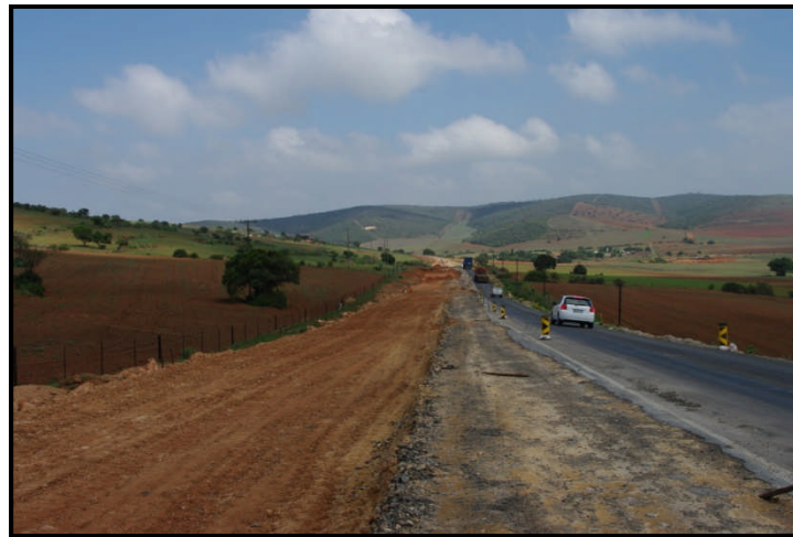
Figure 3: Upgrading of the R72 between Port Elizabeth and Port Alfred
