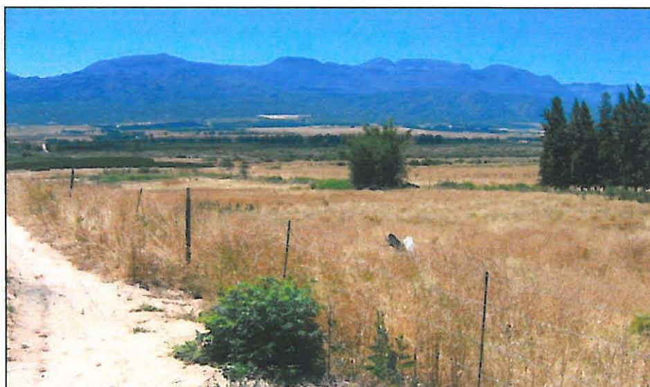
Figure 6: The spillway will run along road at left. The pines mark the approximate middle of the dam
