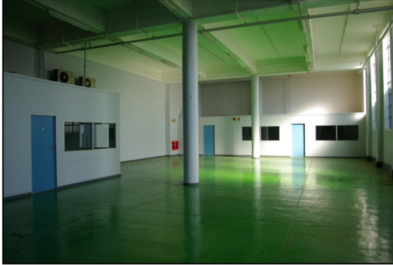
Figure 15: Recent low impact interior alterations to the Historic Period structure
