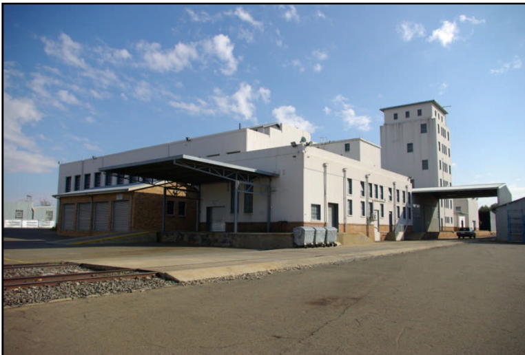
Figure 8: Exterior view of the Historic Period structure
