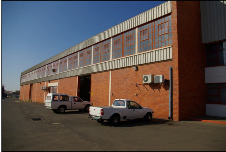
Figure 6: Contemporary Telkom development on the Remainder of Erf 4621
