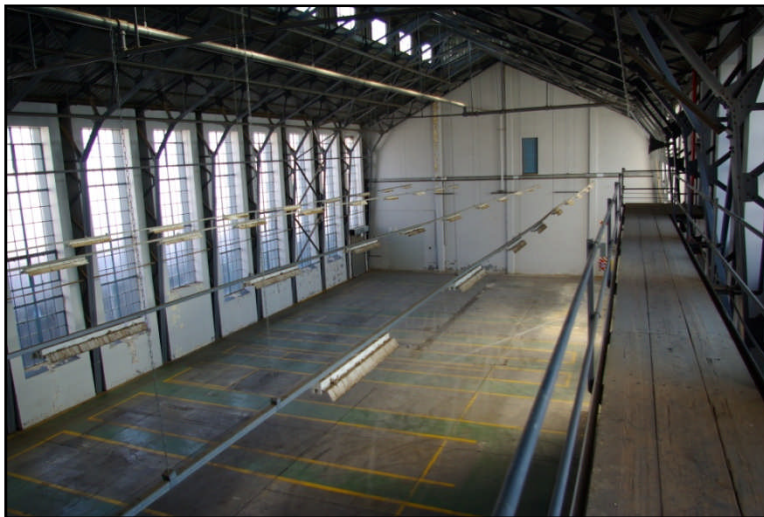
Figure 14: Interior of the Historic Period structure - 2
