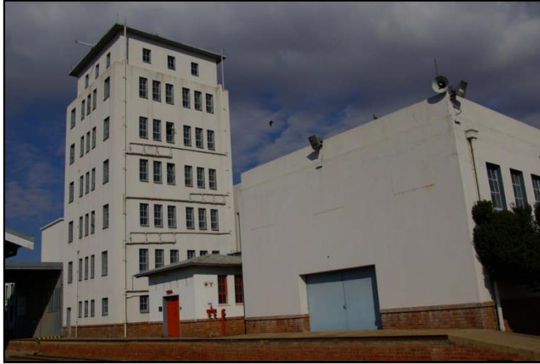
Figure 9: Exterior view of the Historic Period structure - 2
