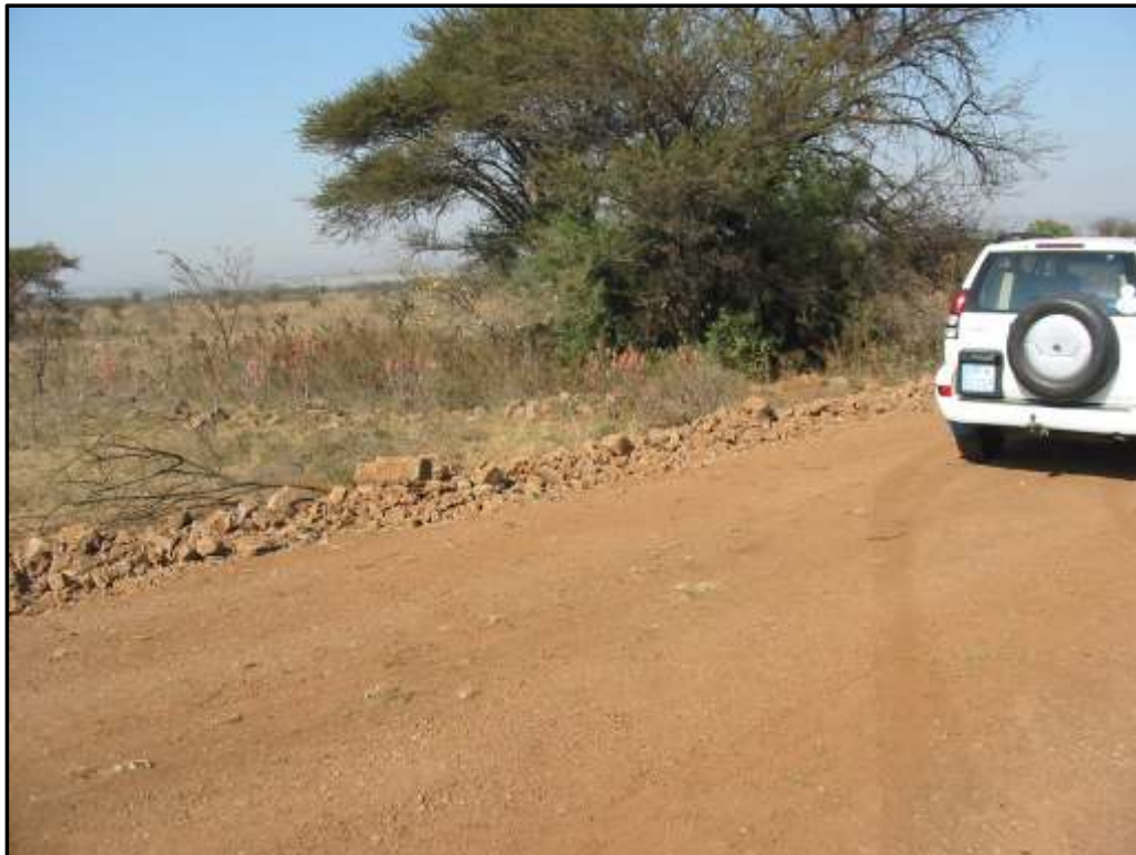
Figure 5: Road through site
