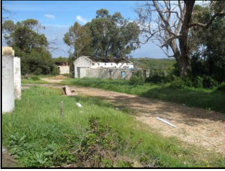
Figure 5. View facing west
