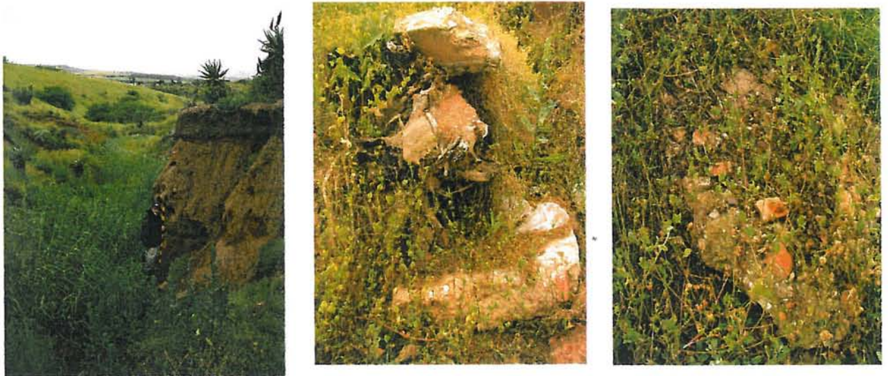
Figure 10: Location of dumped building material and detail
