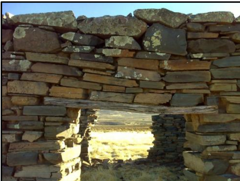
Figure 18. Close-up of the ruins of the main clay packed stone cottage.
