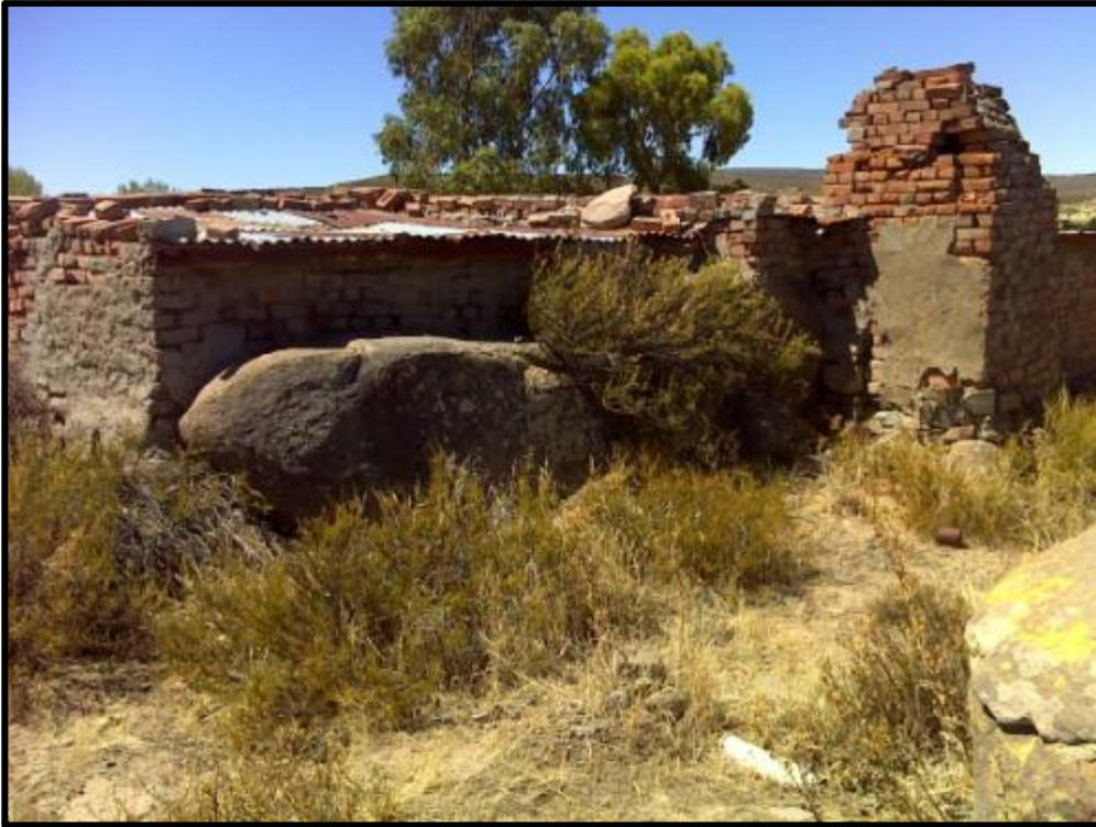
Figure 34. View of the back (left-hand side) of the cottage.
