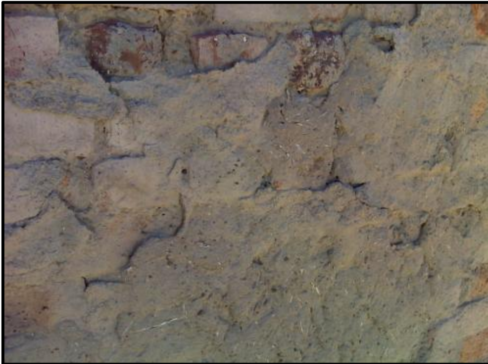
Figure 35. Close-up of the clay/mud packed plastering.
