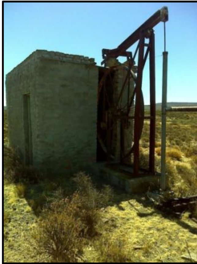
Figure 40. View of the original mill water pump.
