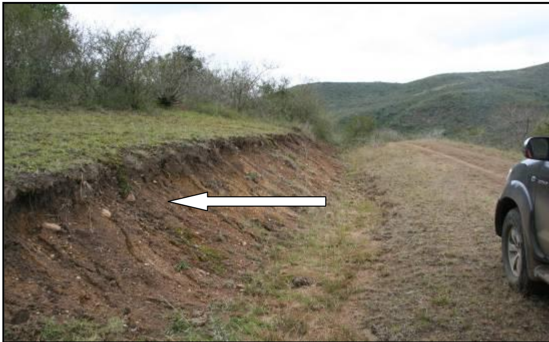
FIG. 13: ROAD CUTTING AT LUS07
