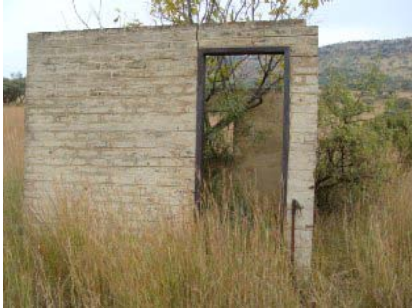
Figure 5: Remains of old building on the property
