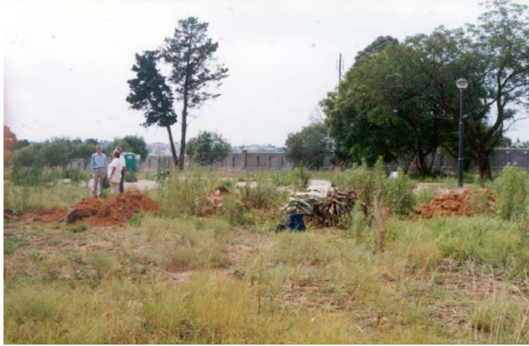
Figure 1. Mound on Honeydew Manor Extension 5 development with three trenches dug through it.
