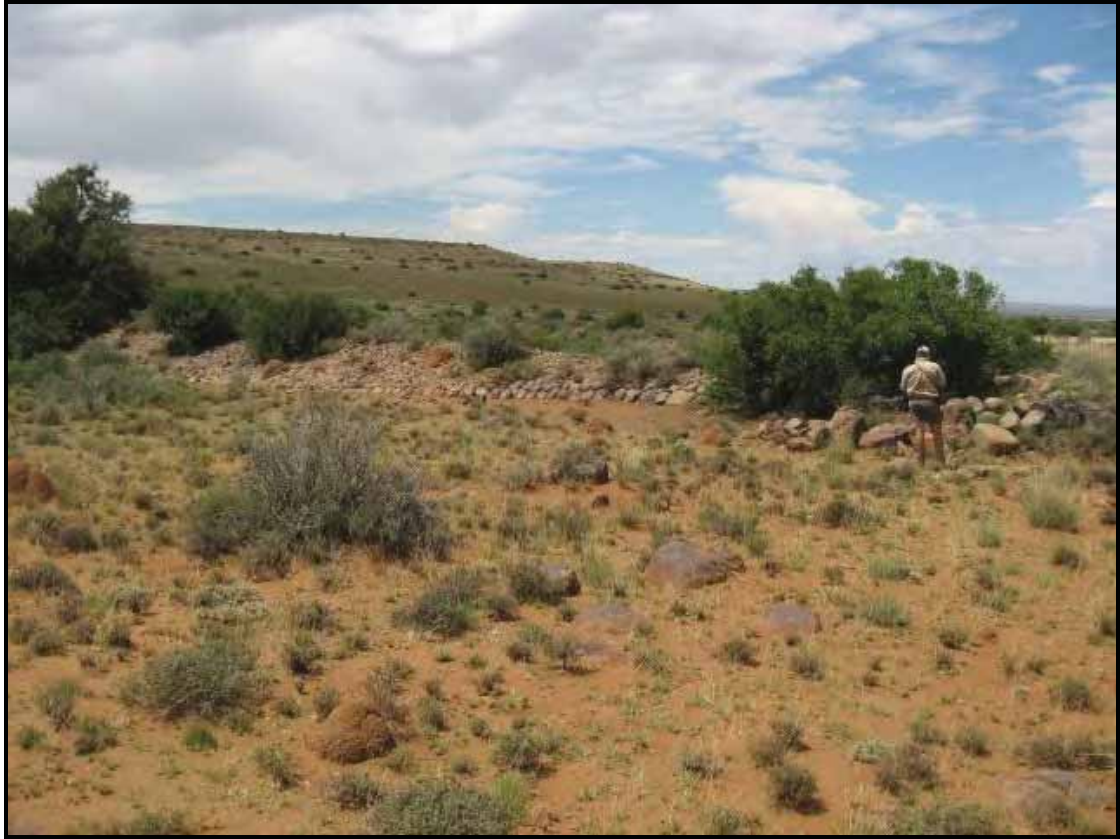
Figure 33 – PH19 – View of dam wall
