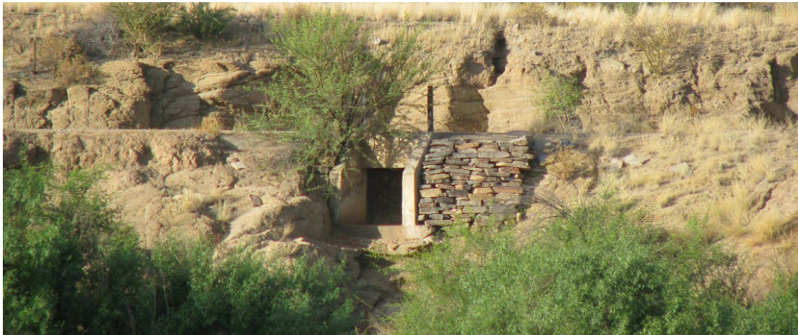
Cement and packed stone strengthening of the old canal. At one point the initials and date “AJK 19-2-1941” are inscribed in the cement.
