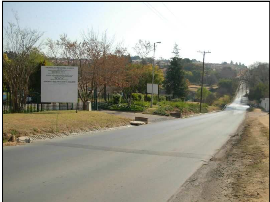
Figure 4: View of low level bridge access from south
