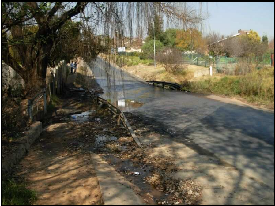
Figure 3: View of low level bridge
