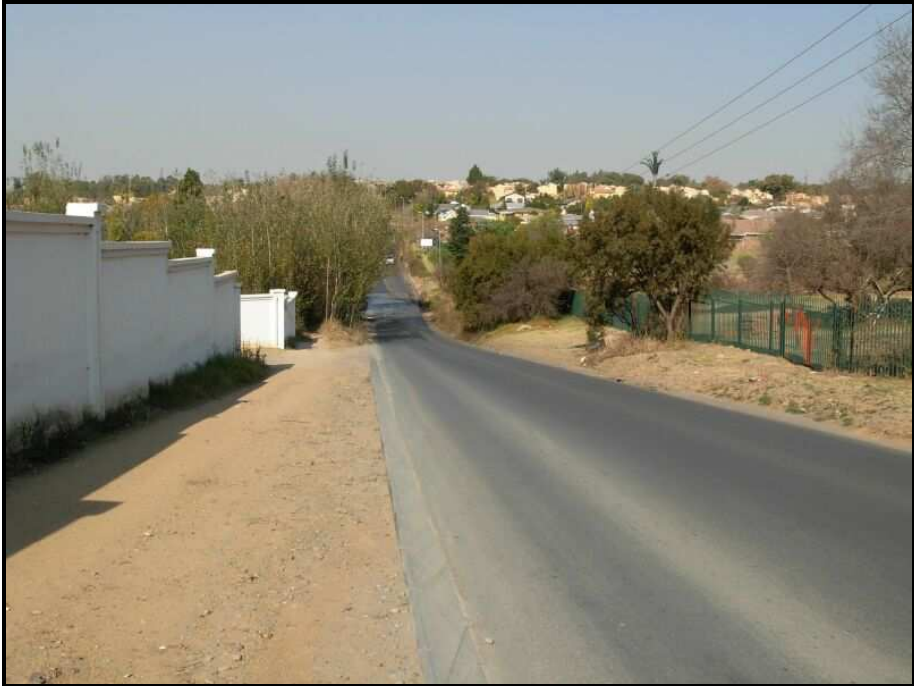
Figure 2: View of low level bridge access from north
