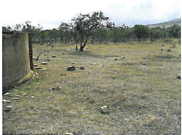
Figure 18. Onverwacht 2 concrete reservoir
