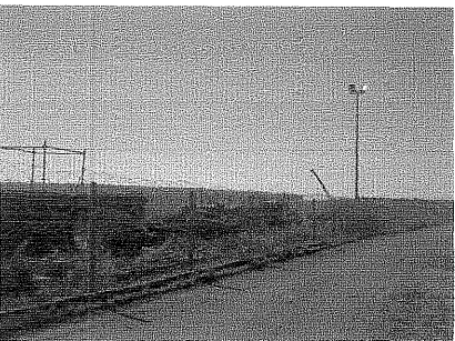
Photo 9: End of proposed pipeline at Injaka Regional Water Treatment Works.
