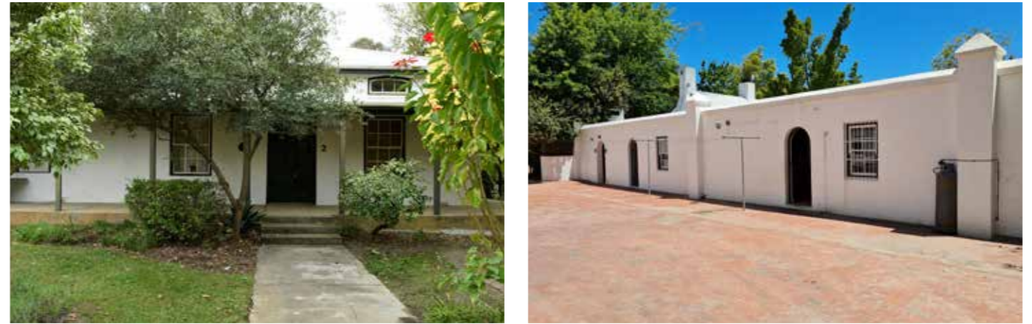
Figure 18. Malherbe House landscaped front garden (Malherbe, 2021), and paved area between the modern service buildings at rear (Fick, 2021)
