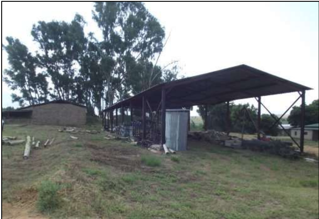
Fig. 38. Site CLB 27. Two sheds, photo looking west.
