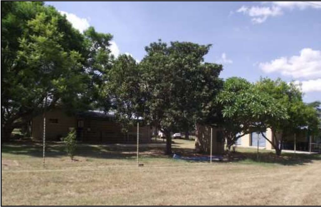
Fig. 35. Site CLB 25. Farm house currently used as animal hospital.
