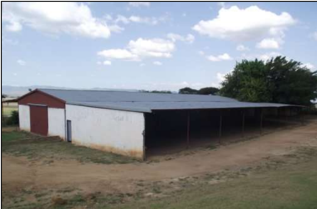
Fig. 36. Site CLB 26. Shed. Photo looking east.
