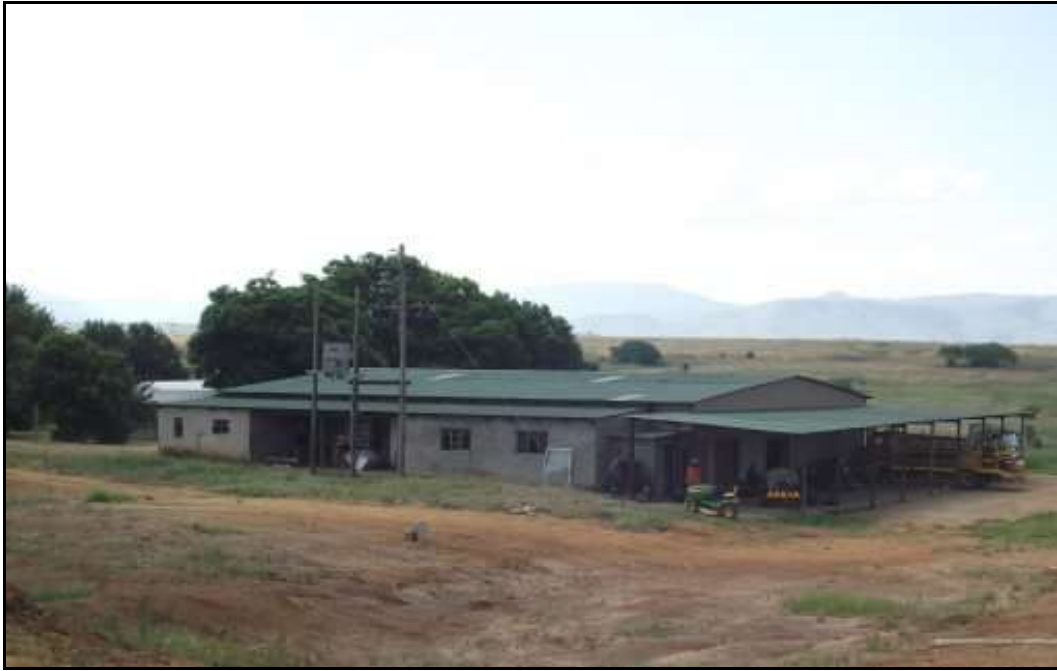
Fig. 39. Site CLB 27. Working farm shed.
