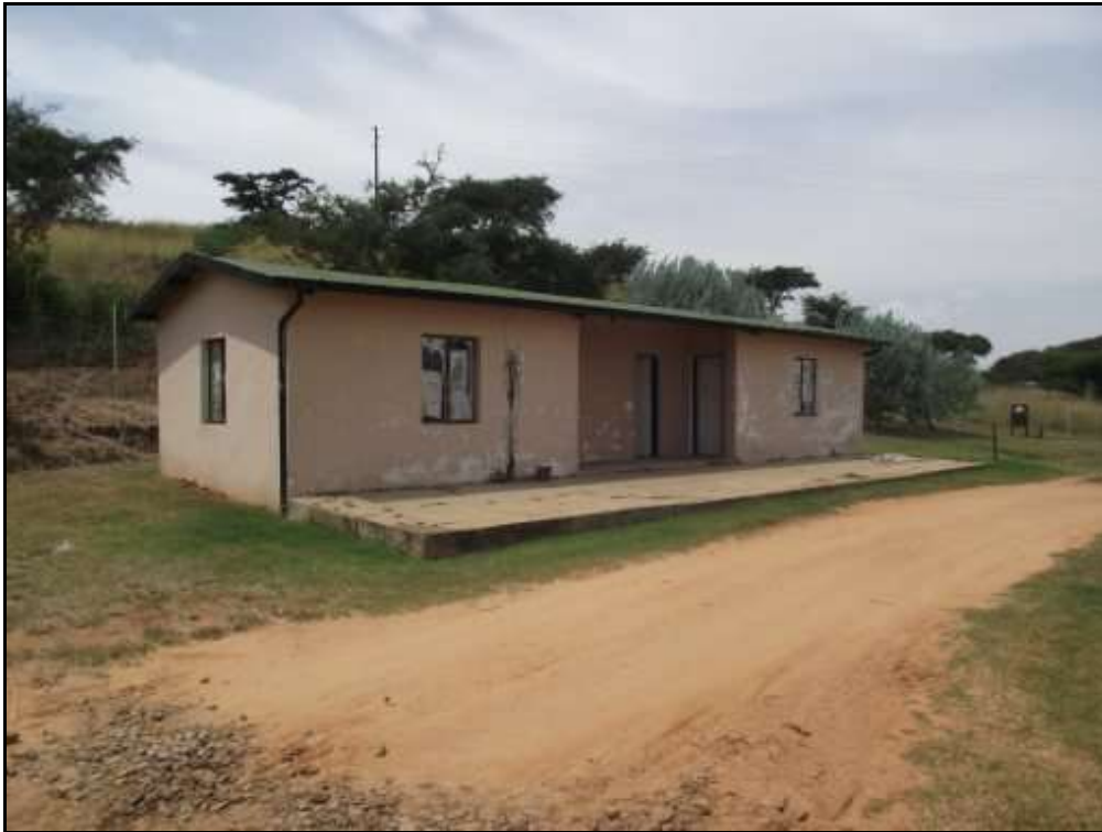
Fig. 15. Site CLB 11. Dressing rooms and toilets.
