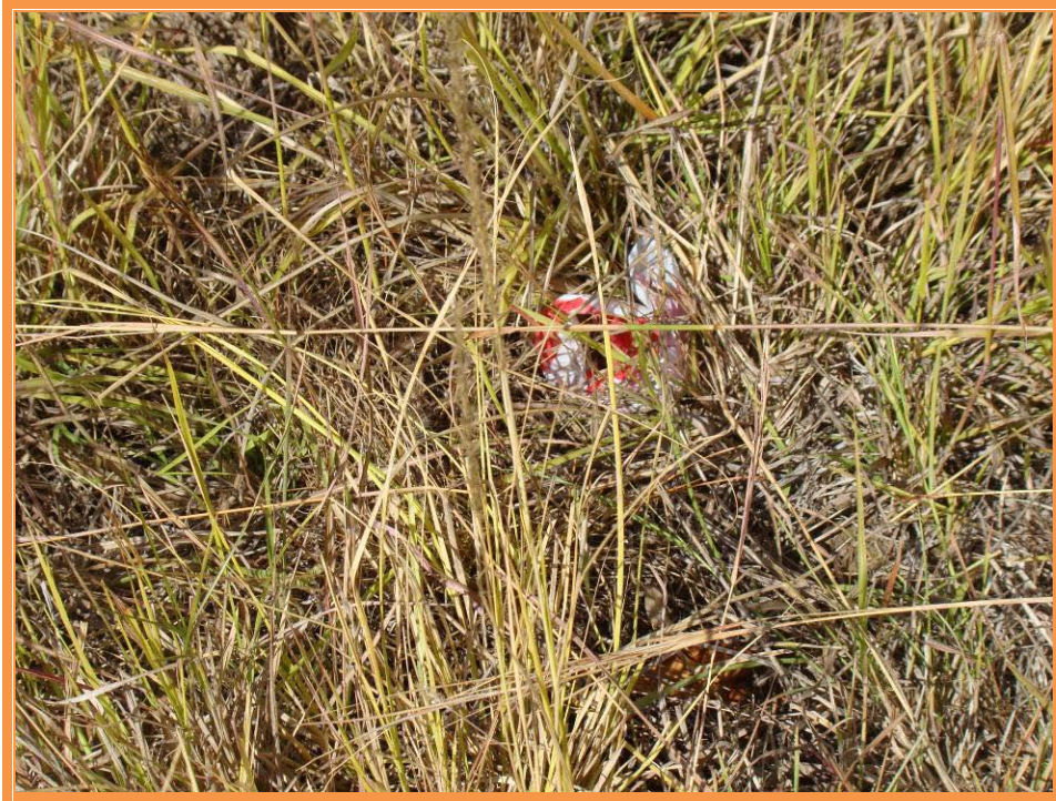
Plate 2: The powerline route is clearly marked by iron pegs with red tape indicating the position of proposed poles. Grass cover on some portions is dense limiting total ground surface inspection.
