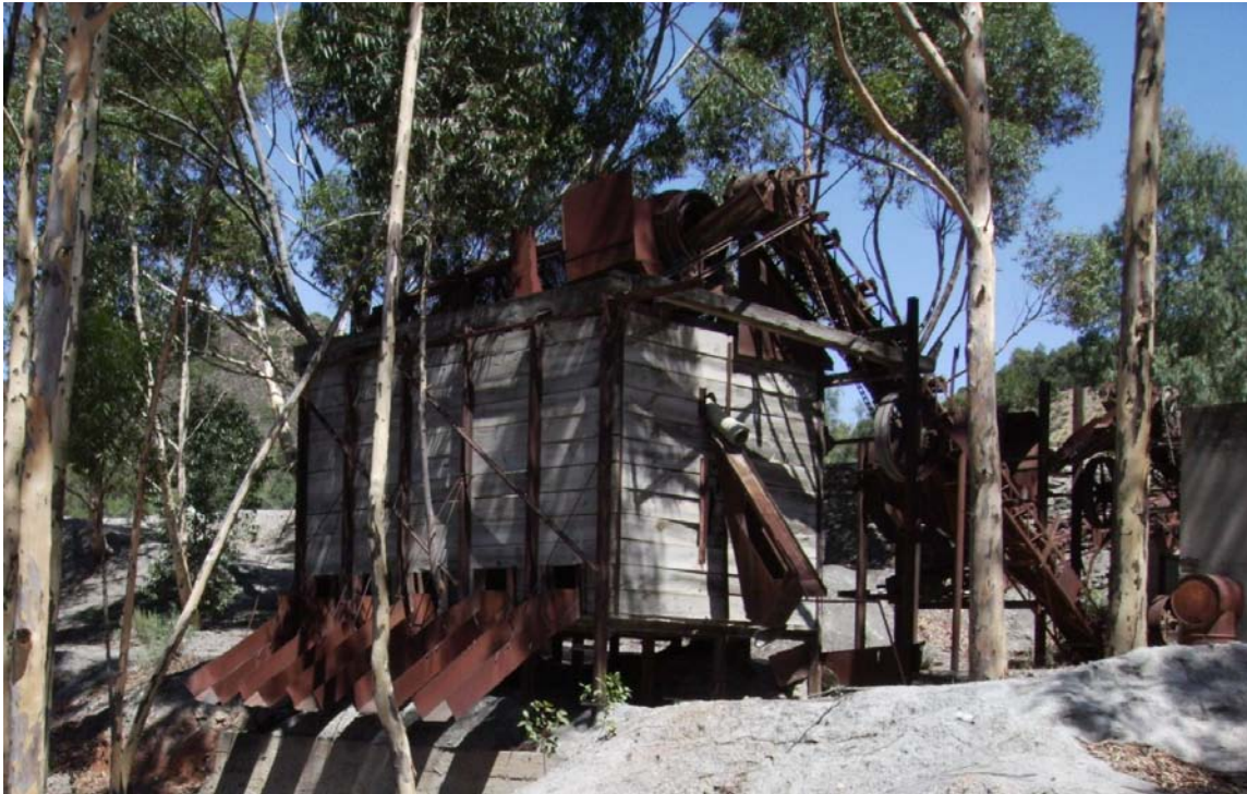
Figure 6. The museum preserving the old crushing plant – an industrial artefact.
