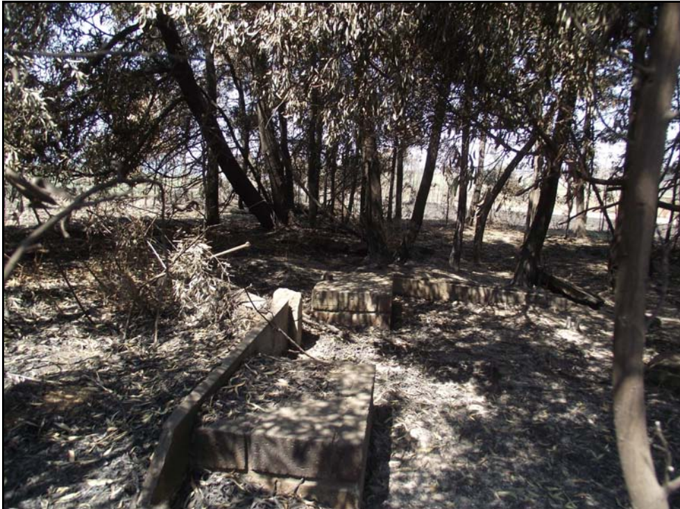
Fig. 9. Site WK 5. Small retaining walls.
