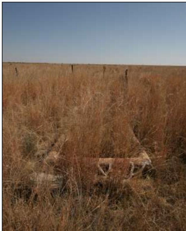
Figure 15: Semi-formal dressing built with local stone and cement.
