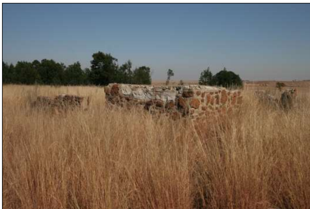
Figure 9: General view of building
