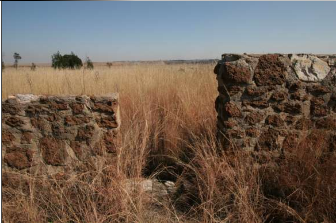
Figure 10: View of possible doorway, note cement mortar used.
