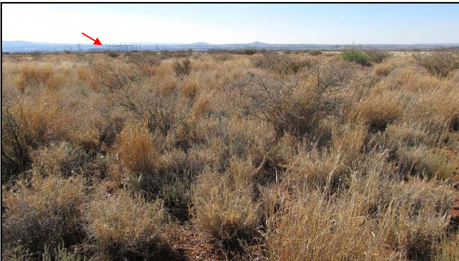
Figure 9. View of the site facing north. Arrow indicates the Burchell substation
