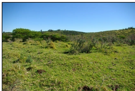
Figure 40: Overgrown structure foundations associated with G6
