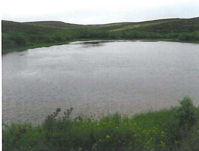
Figure 3. The Klawervlei Dam facing west
