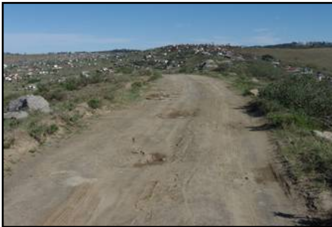
Figure 7: View of the northern part of the KwaThuba road study site
