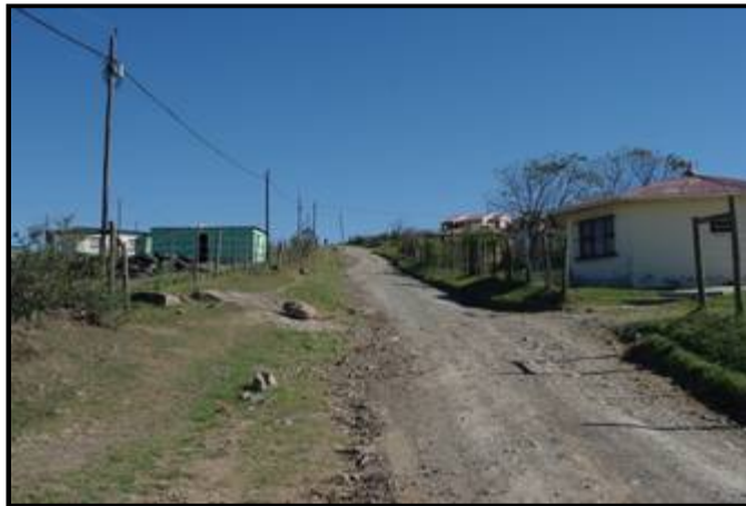
Figure 6: General view of the existing road through KwaThuba Village
