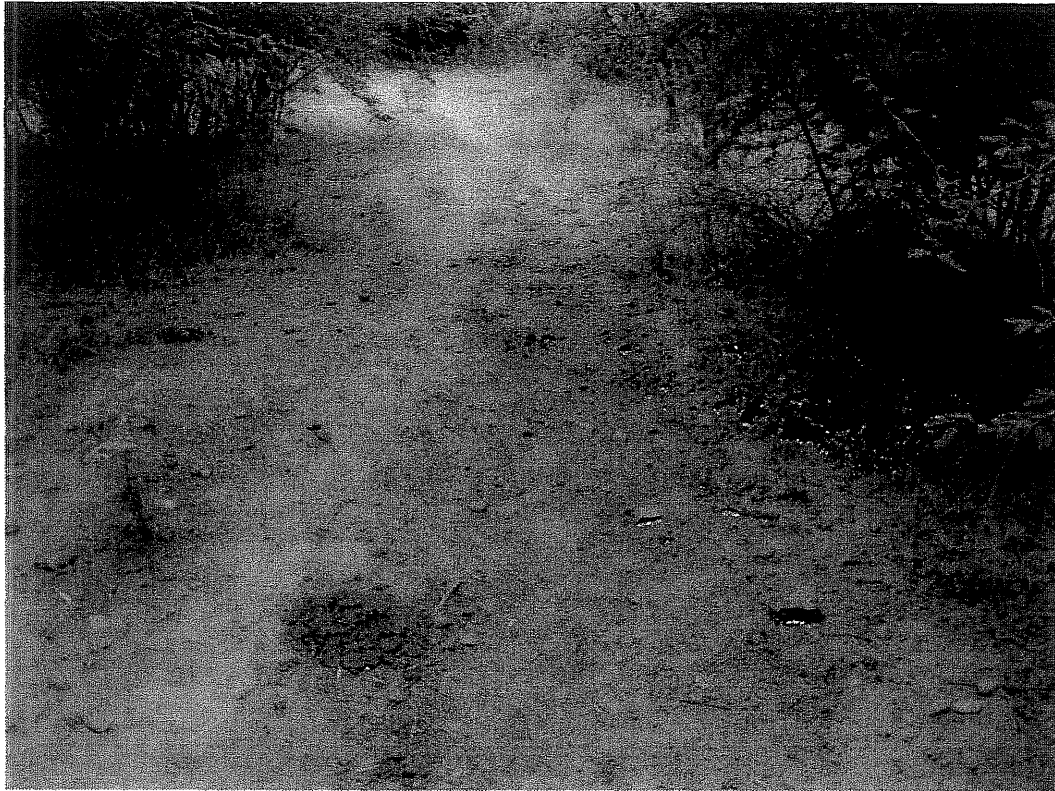
Photo 9: LKV 001. Eroded pathway.
