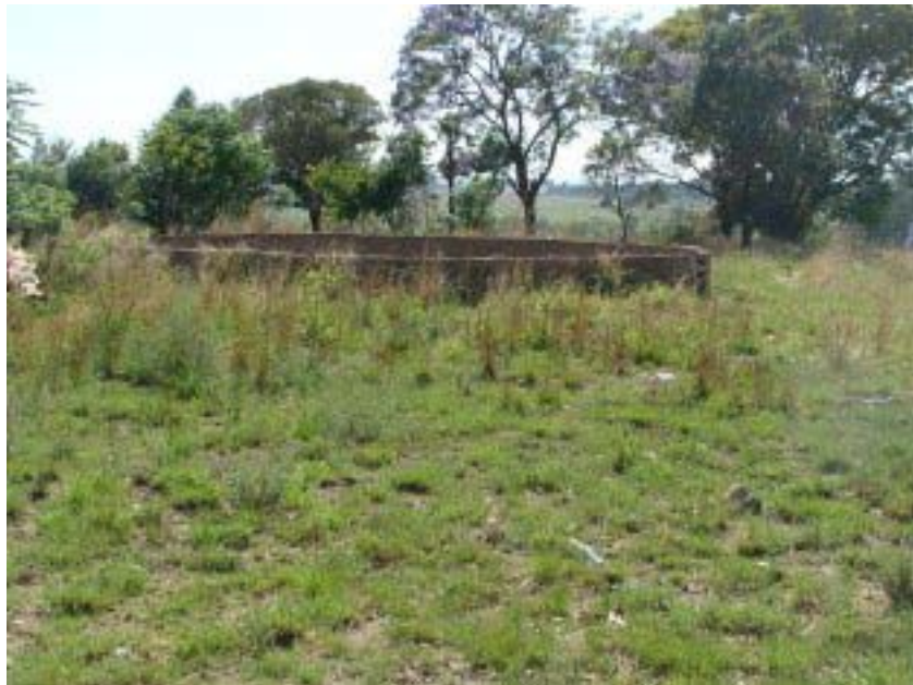
Figure 7: Remains of an old cement dam in the area.
