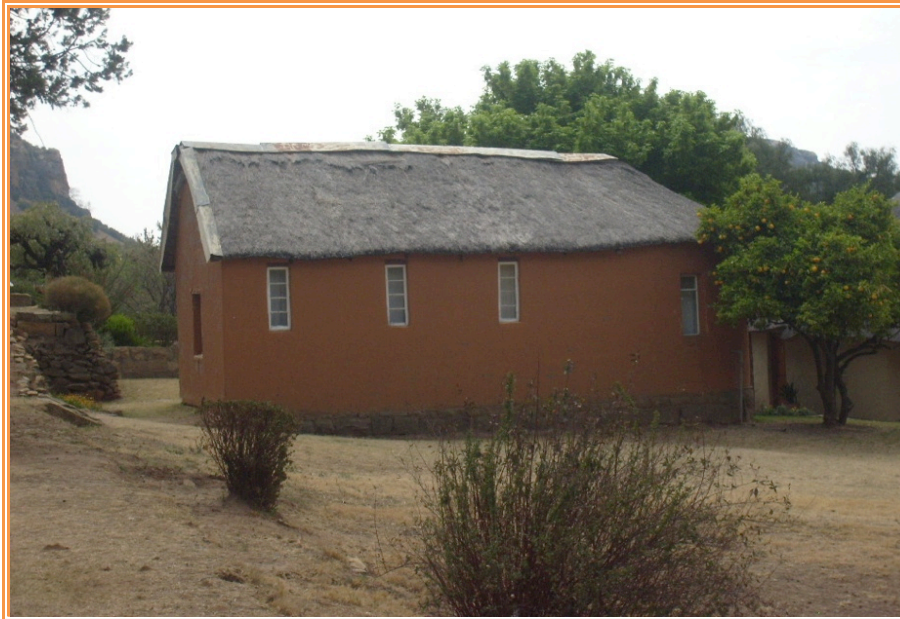
Plate 1: View of an old church building at St Augustine Priory.
