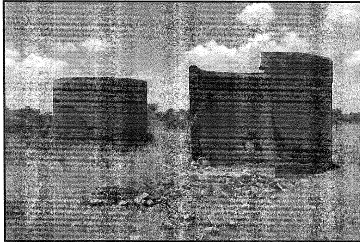
Figure 46: Two water towers at Site HS1
