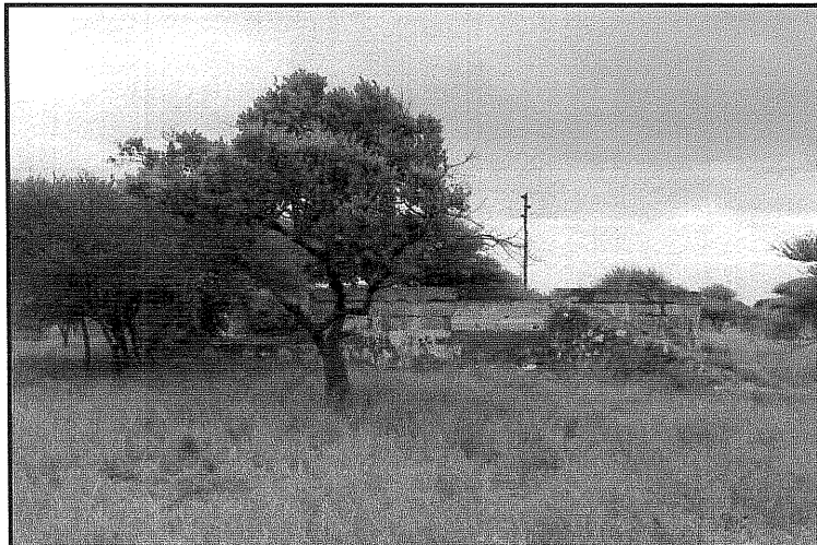
Figure 18: The dam located in close proximity to the residence and forming part of Site HR1
