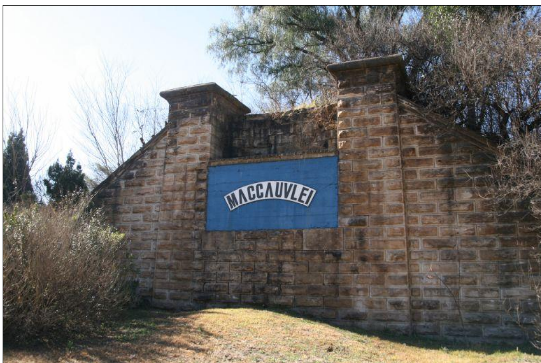
Figure 14 – Stone bridge foundation of RW1
