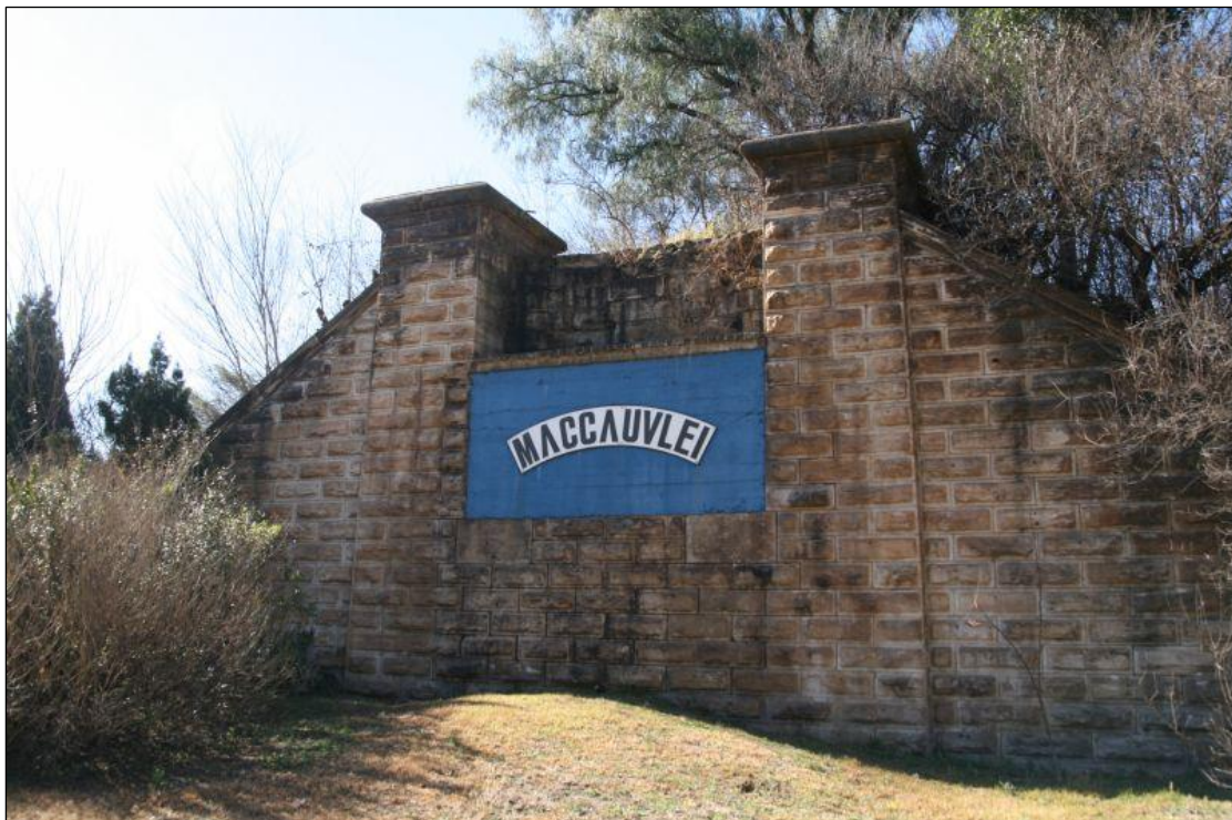
Figure 6 – Old bridge foundation close to where proposed crossing to the Gauteng Province over the Vaal is (Site RW1)
