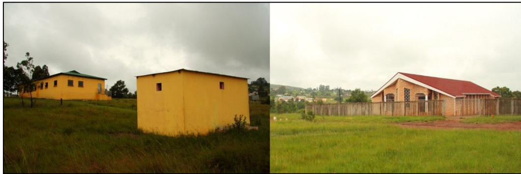
Figure 6: Church buildings on the northern extremity of the survey area.
