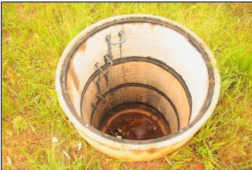
Figure 4: Concrete manholes occur across the survey area.
