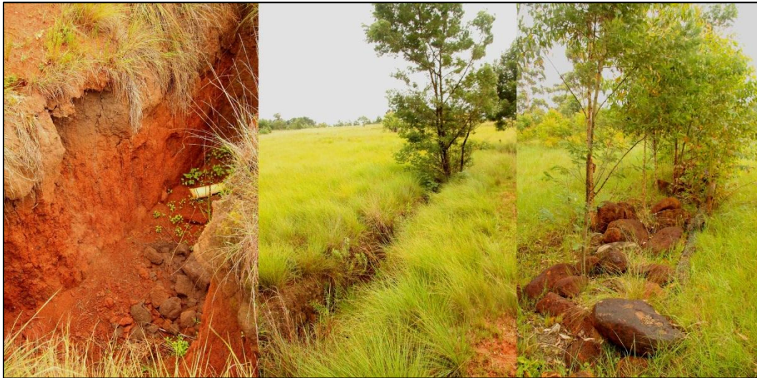
Figure 5: Erosion gullies, excavation trenched and stone-filled ditches at the Libode site.
