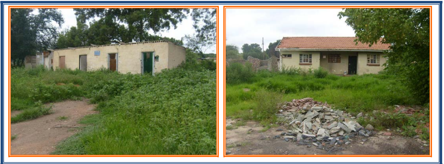
Plates 5 and 6: Abandoned buildings within the alternative site A.
