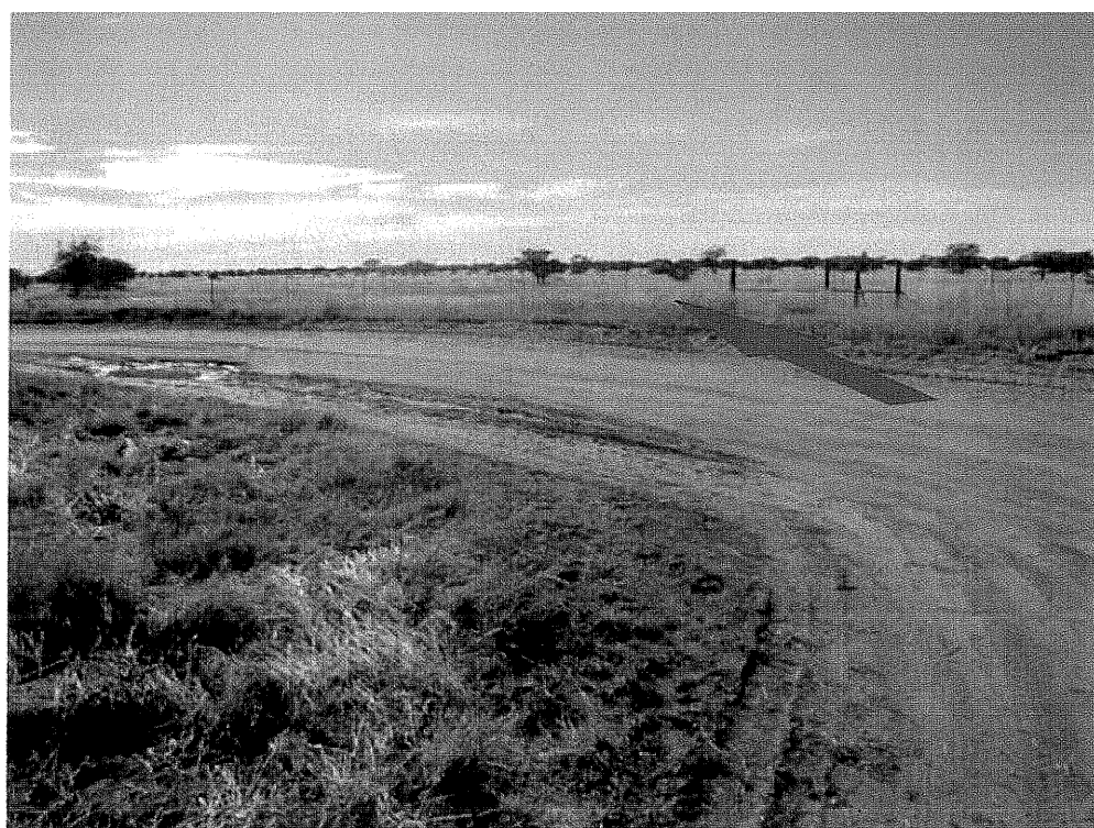
Figure 5. Section A to B. The pipeline cuts through 1 km of undeveloped veld (above) and terminates at a road junction.
