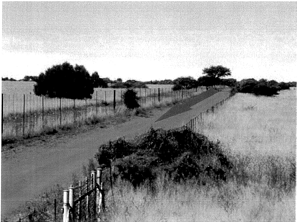
Figure 6. Section B to C. The pipeline will be placed alongside an existing farm road.
